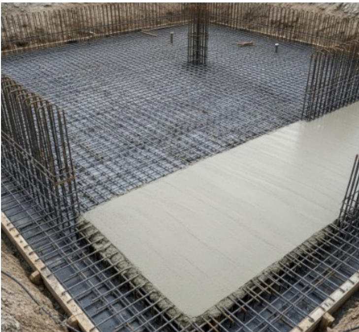
Fig. 4 Square raft foundation
