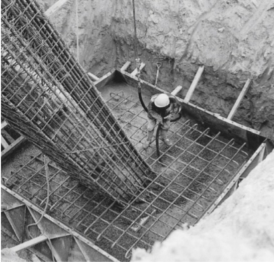
A- Pad & chimney foundation
