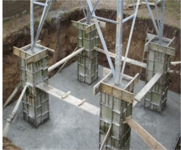
B- Concrete mat foundation
